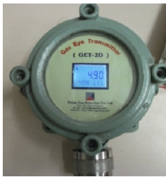
Gas Detector Unit with Display
